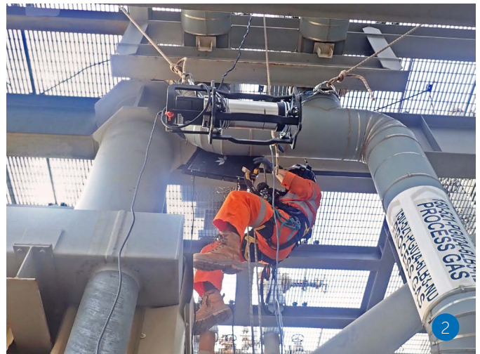
After removal of insulation by Kaefer onsite team.
